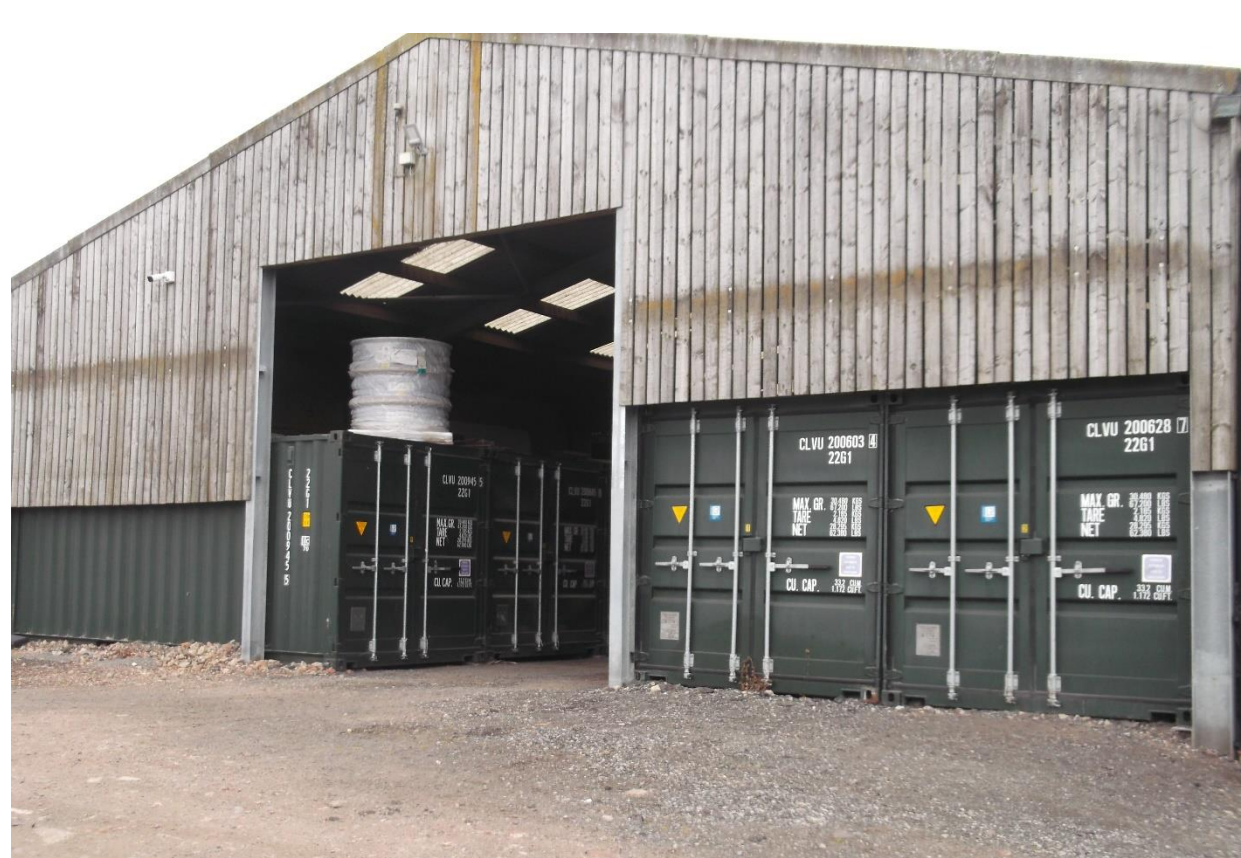
Containers in situ within building
